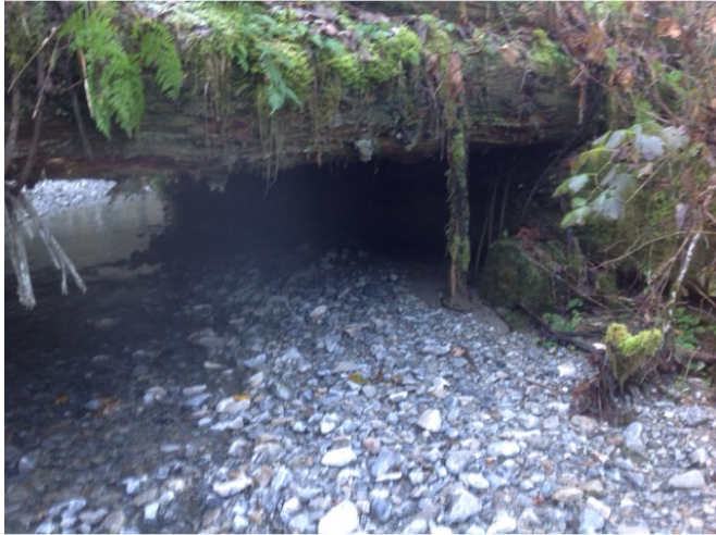
Left Bank Abutment when facing downstream
