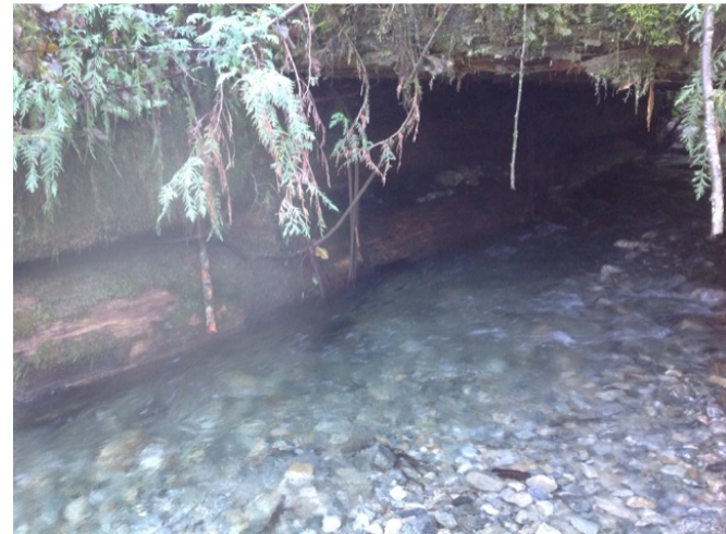
Right Bank Abutment when facing downstream
